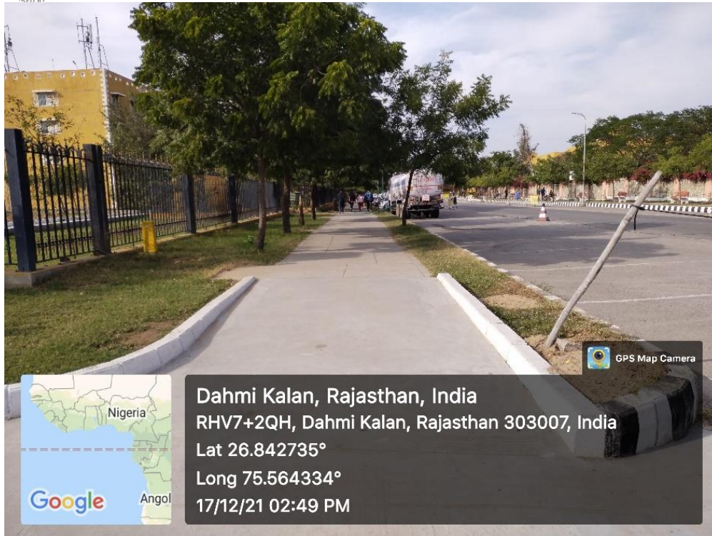
Picture 6: Sidewalks have curb cuts and ramps for individuals with disabilities
